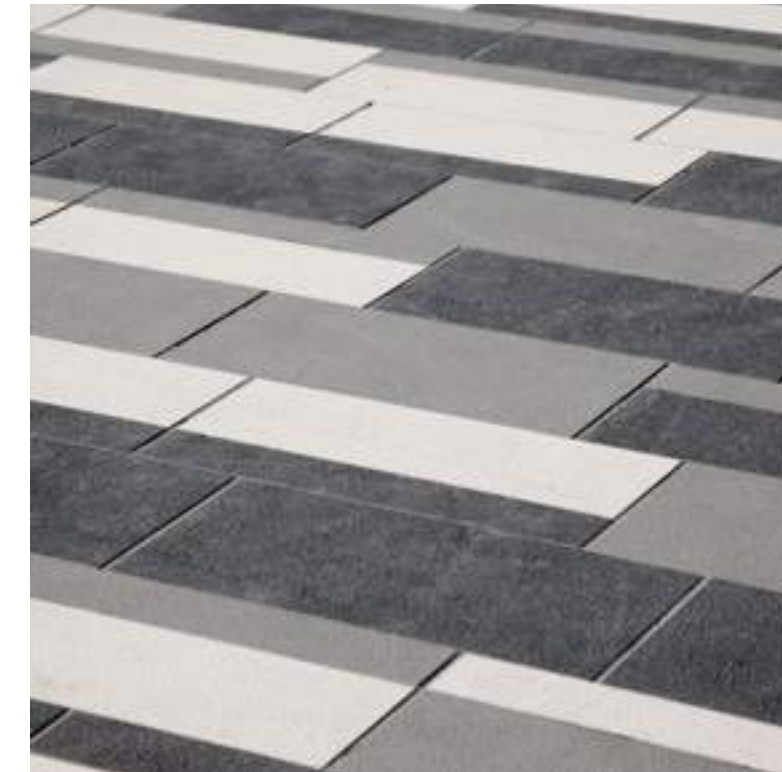
MAIN ENTRANCE PAVING
