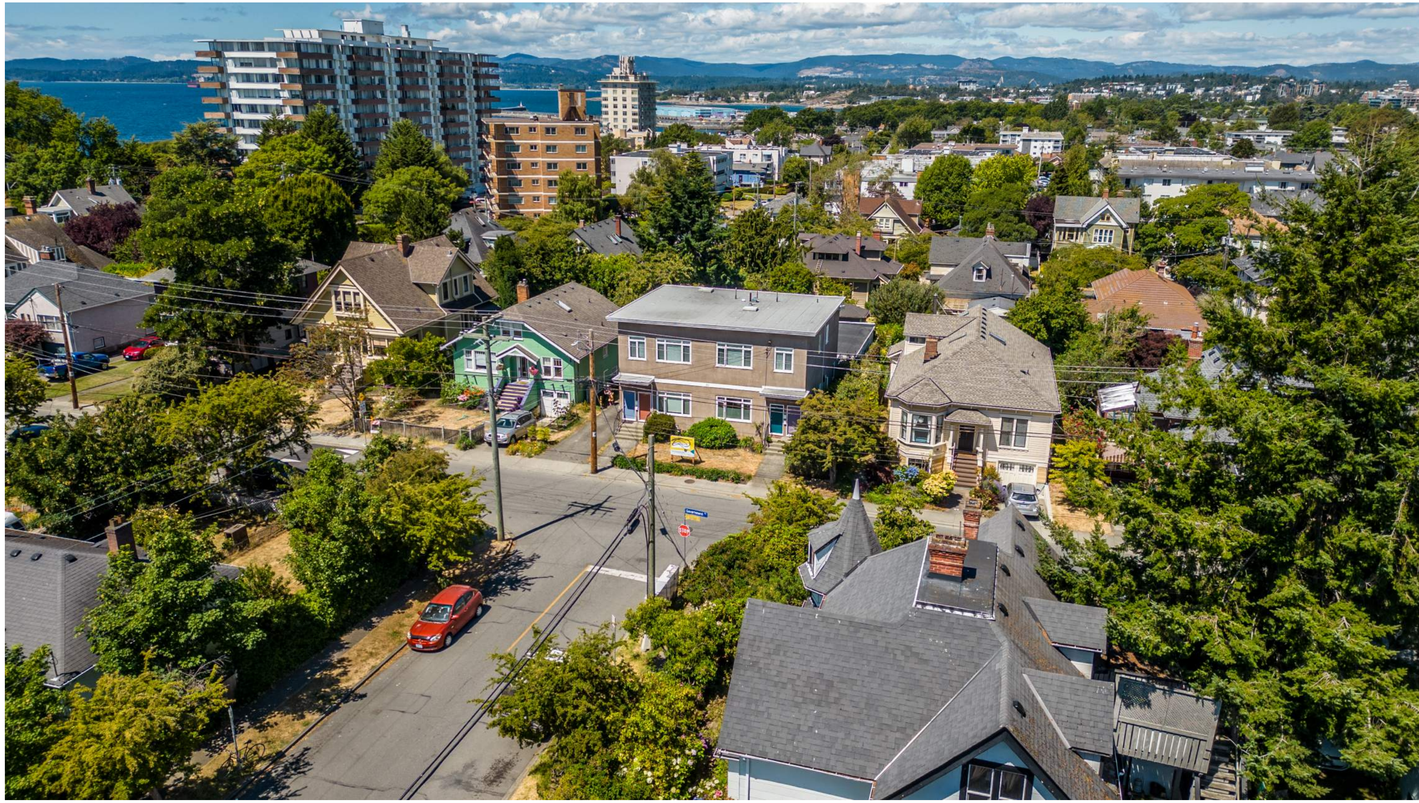
Existing Building, 50 Government
