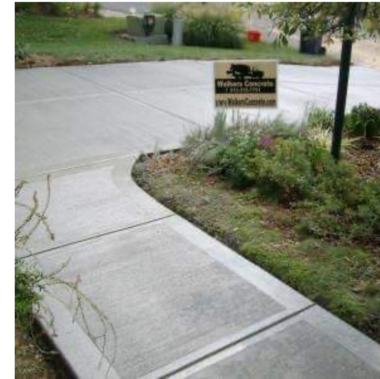
CIP CONCRETE PAVING
