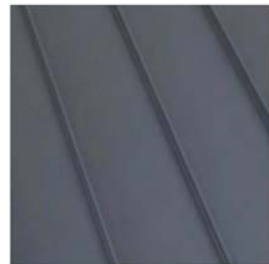
STANDING SEAM METAL ROOFING
