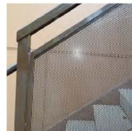
HANDRAIL & GUARD WITH PERFORATED METAL PANEL
