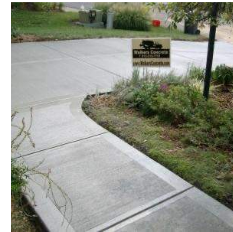
CIP CONCRETE PAVING
