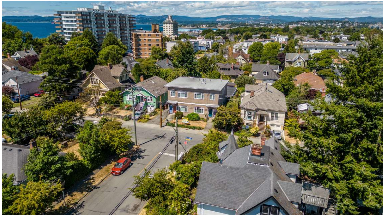
Existing Building, 50 Government
