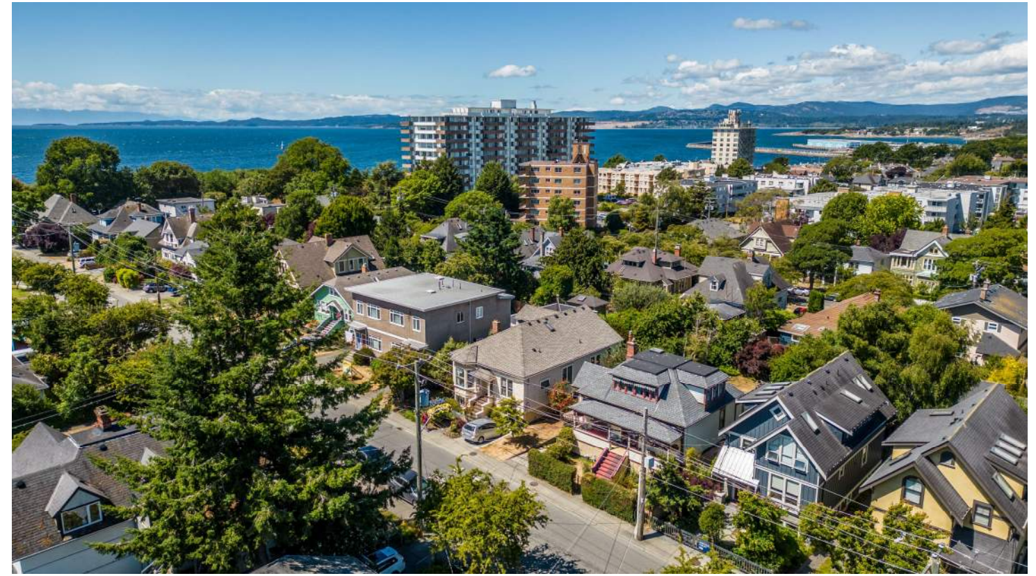
Existing Building, 50 Government
