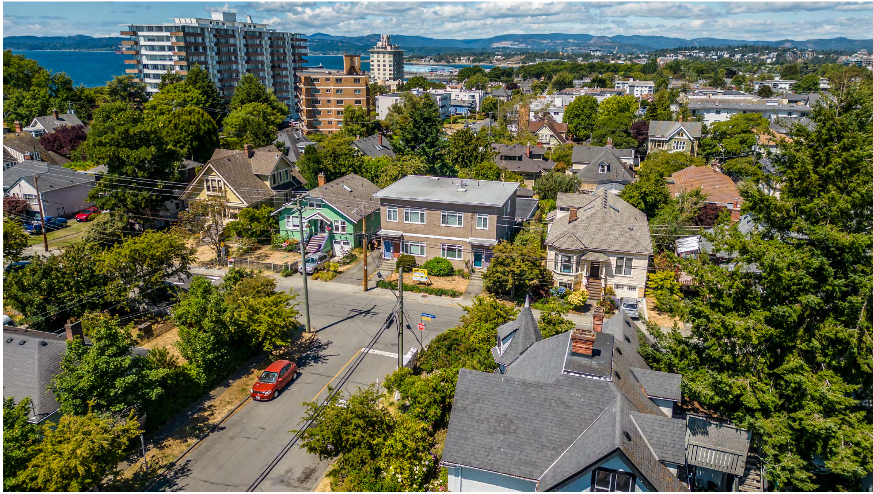
Existing Building, 50 Government
