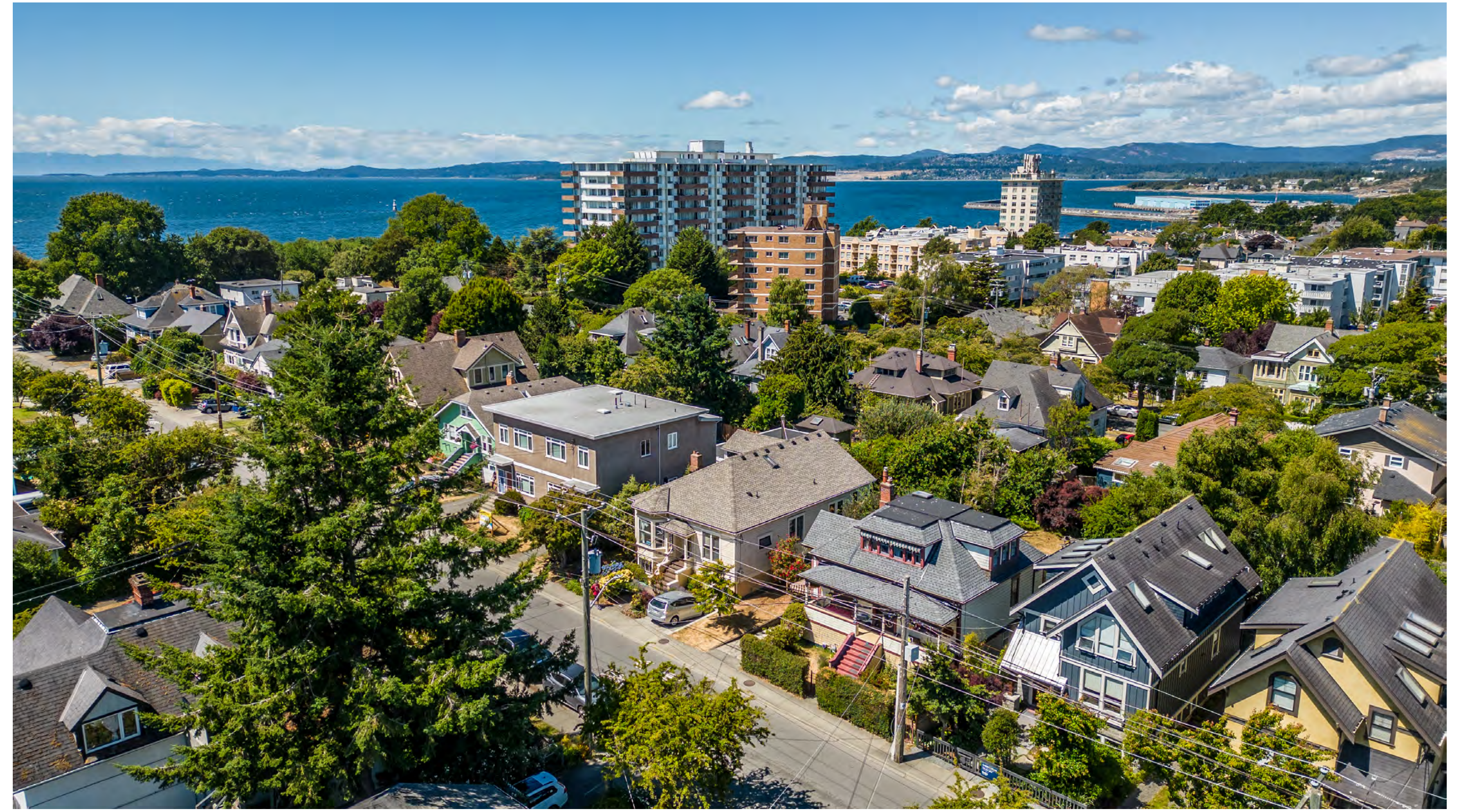
Existing Building, 50 Government
