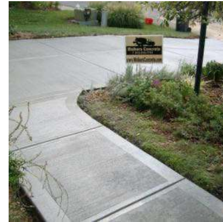
CIP CONCRETE PAVING
